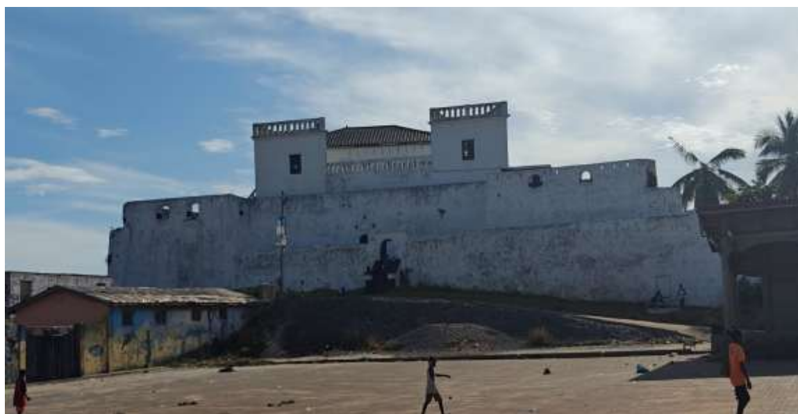
Photo 7: Fort St. Antonio, Axim (Nzema East District).
